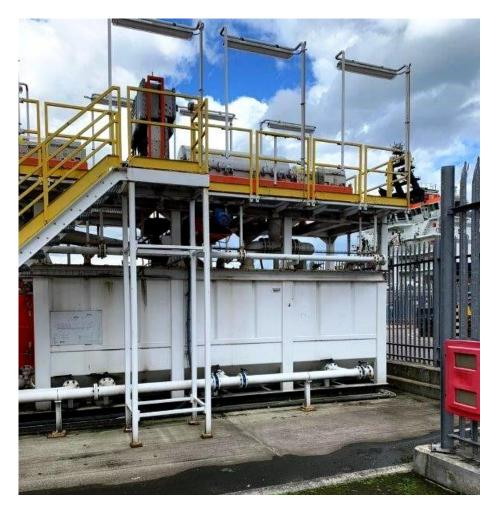
Customised steel structure, these stands are split into section and can be easily assembled once delivered on the site.
